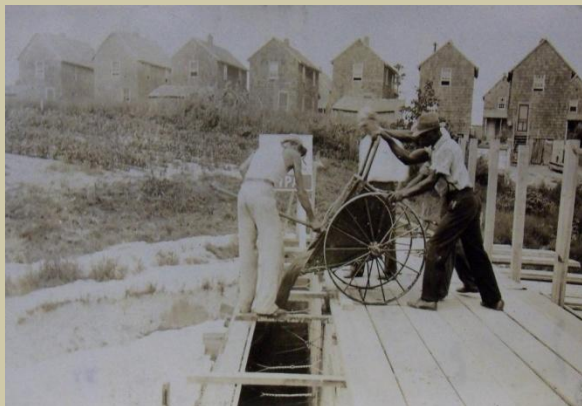
( Left: Workers pouring concrete for the Johnson's Pond Dam, 1936. Photo by the WPA, provided courtesy of the University of Maryland College Park Archives. Right: Johnson's Pond today. Part of the top of the dam can be seen at the far end of the pond. Photo taken by Brent McKee, 2011)
